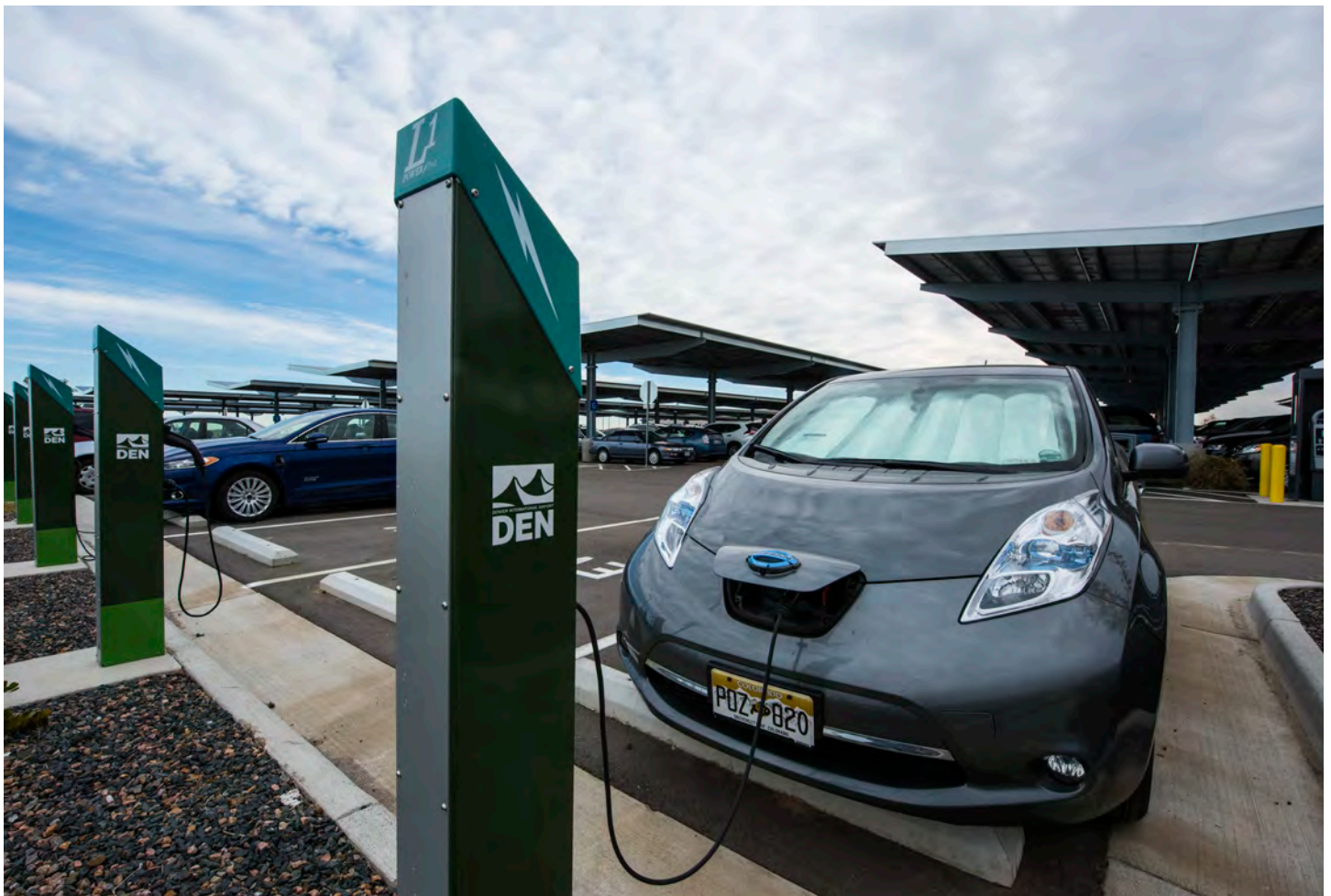
This electric vehicle charging station is powered by solar panels installed on a parking canopy. Because electric vehicles can be powered by clean energy sources including wind and solar power, they can enable a transition to a zero-carbon transportation future. Credit: Dennis Schroeder, National Renewable Energy Laboratory
